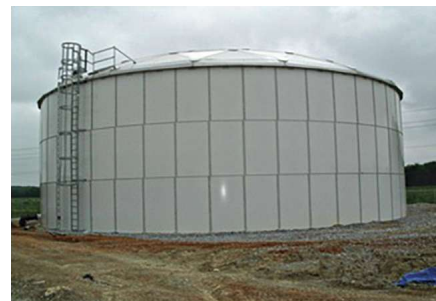
FIGURE 4 Fire protection water storage tank.
