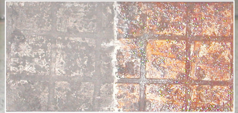
After Applying Vapro 812
